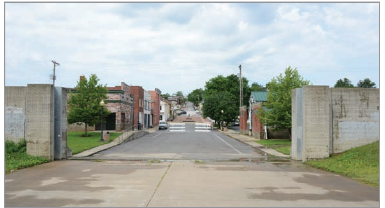
Floodgates in the levee at the base of Hill Street, open . . .
