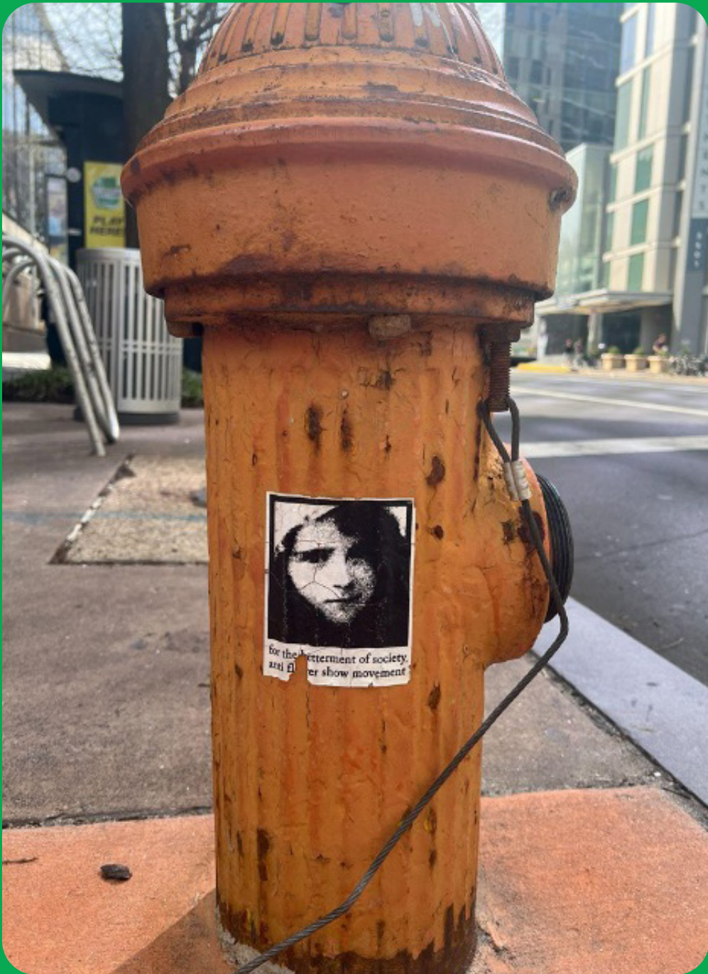
↑ AFSM sticker on a fire hydrant. Photo by Danny Jarabek.
