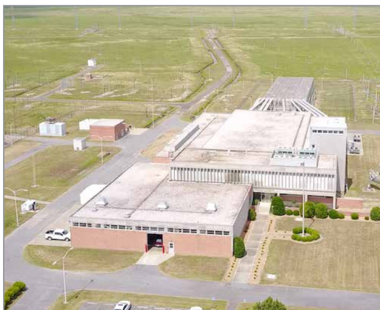
Transmission Station B, Greenville, North Carolina.
