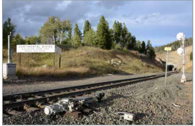
Railway tunnel under/over the Divide at Mullan Pass.
