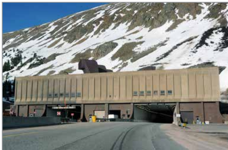
The west portal of the Johnson and Eisenhower Tunnels, carrying Interstate 70 over/under the Divide. CLUI photo
