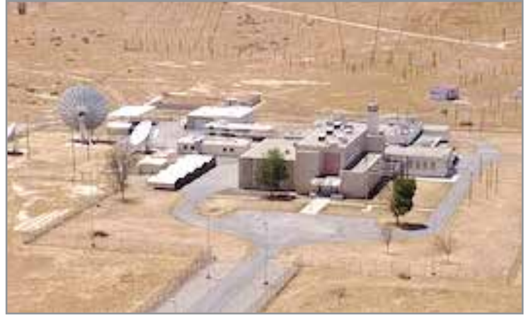
Delano Transmission Station, Delano, California.
