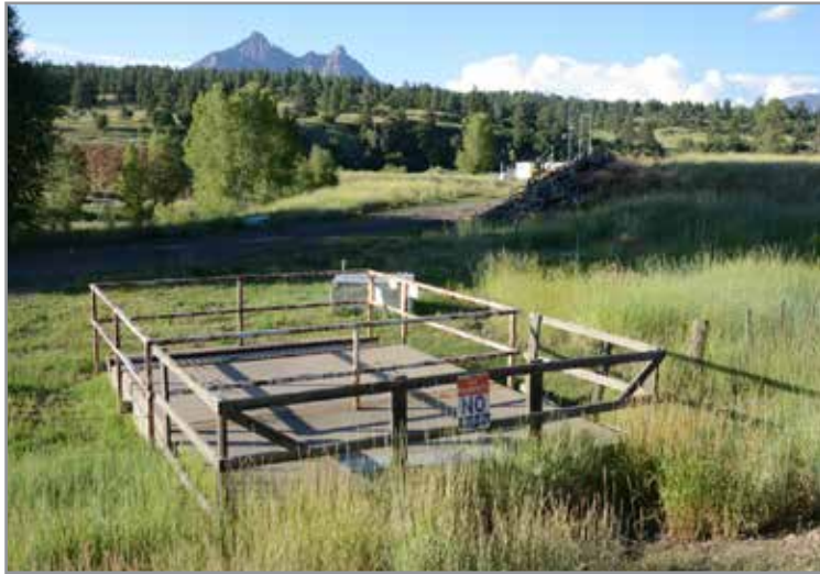
The access hatch to the Azotea Tunnel, as it leaves the Oso Diversion Dam, taking Colorado River water south into New Mexico and to the Rio Grande, crossing the Continental Divide along the way. CLUI photo
