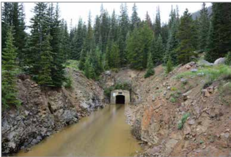
The east portal of the Twin Lakes Tunnel.
