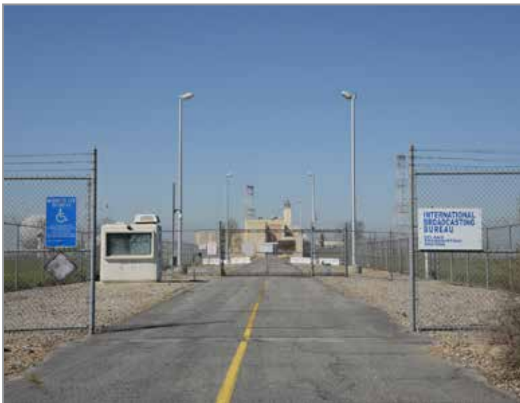
The entrance to the former Delano transmission station.
