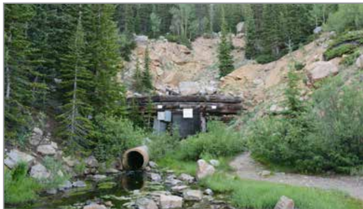
The Busk-Ivanhoe Tunnel, a former rail tunnel converted to a car tunnel, now just carries water, in a pipe over the Continental Divide. CLUI photo
