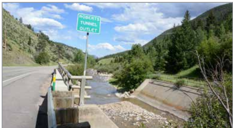
The east portal of the Roberts Tunnel, flowing into the North Fork of the South Platte River.
