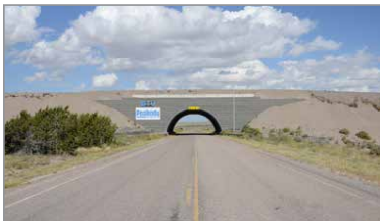
The haul road bridge, which connects the two parts of the El Segundo mine, travels over the highway that divides it, on the Continental Divide. CLUI photo
