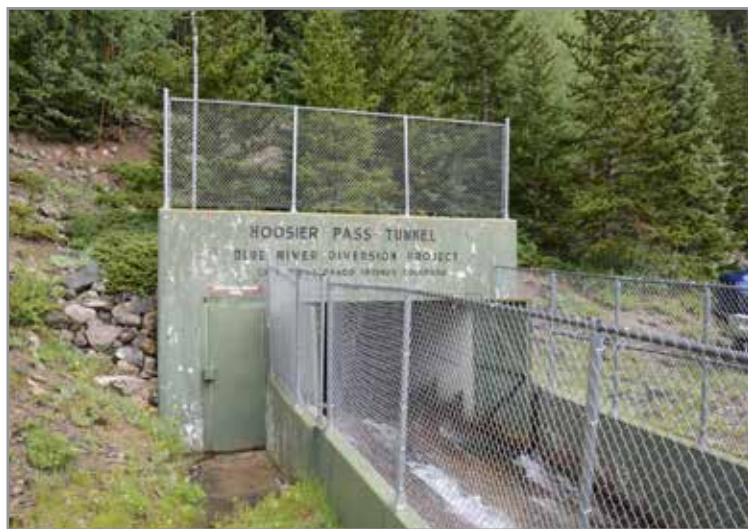
The Hoosier Pass Tunnel, emerging from under the Continental Divide. CLUI photo
