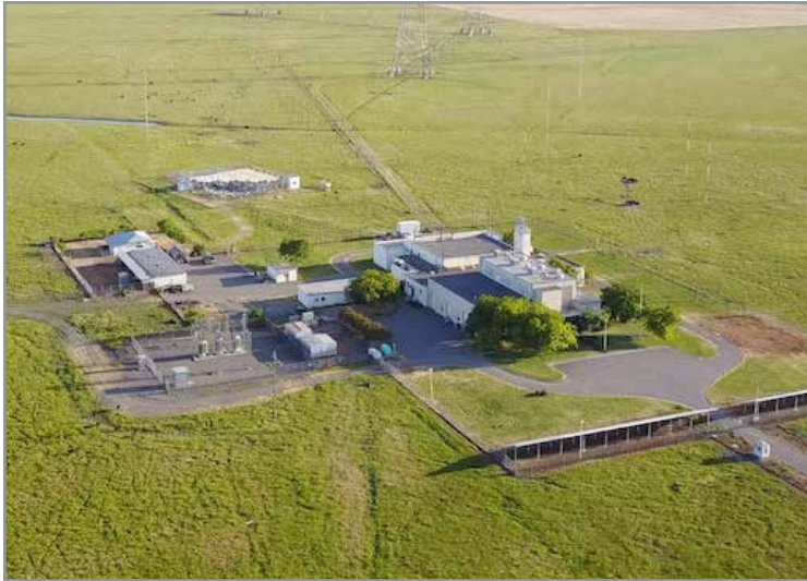
Dixon Transmission Station, Dixon, California.
