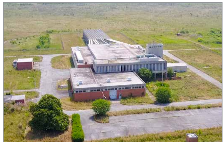
Transmission Station A, Greenville, North Carolina.
