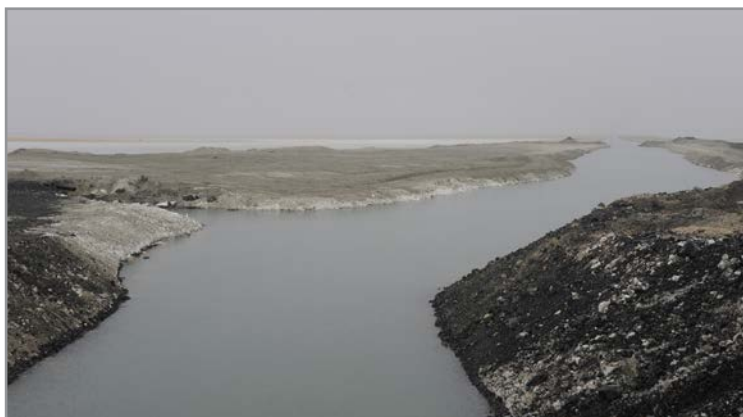
The beginning of the Behrens Trench, where concentrated brine from the impoundments at Clyman Bay travels in an inclined subaqueous trench across the bottom of the Great Salt Lake, to a potash plant on the other side. CLUI photo
