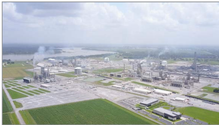
The CF Industries plant in Donaldsonville, Louisiana is the largest single source of nitrogen fertilizer in the nation, by far. Unlike potassium and phosphorus, which are mined from solids in the earth, nitrogen fertilizer is made into a solid (and liquid) out of natural gas, extracted from the earth. CLUI photo
