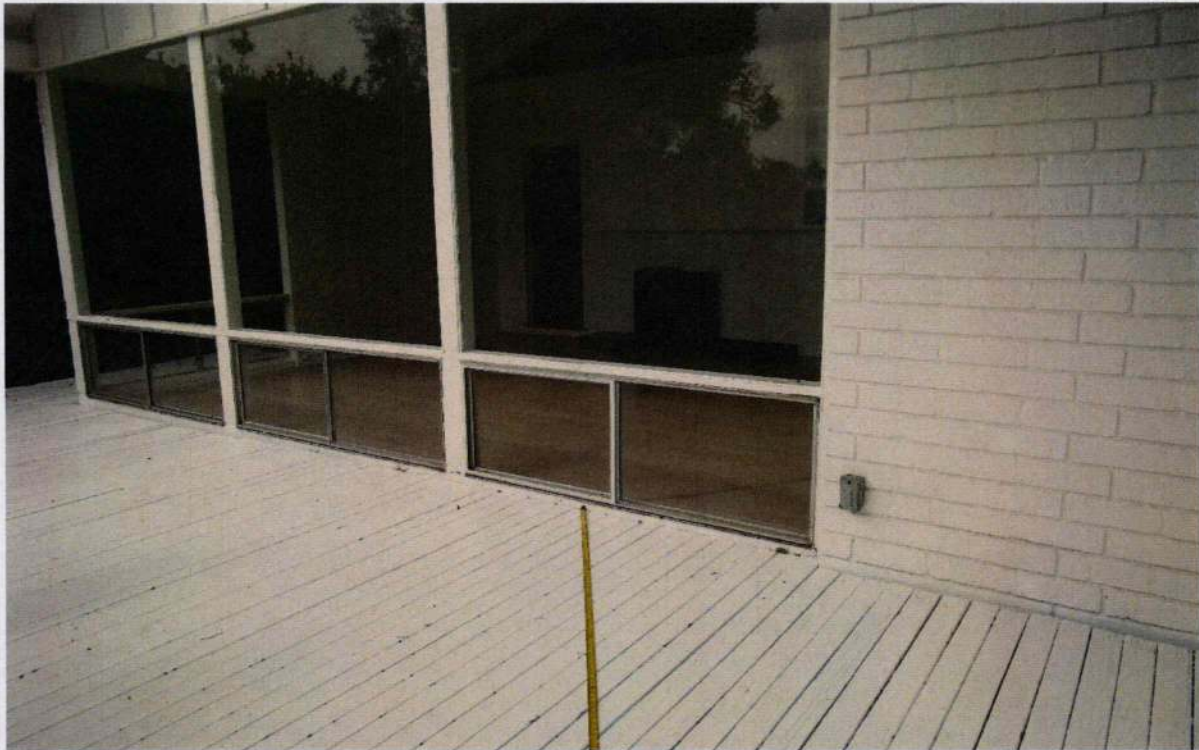
Exhibit 2A: The primary view was documented from an exterior location, ten feet from a primary living area
