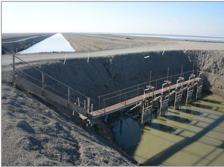
Intersecting canals at the end of the Kings and Tule Rivers, on Tulare Lake. CLUI photo
