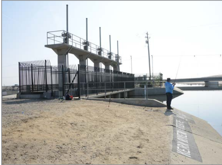
The gates of the Kern River Intertie, where the Kern River meets the California Aqueduct. CLUI photo
