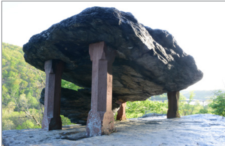
Jefferson Rock. Sometime in the late 1850s, the armory superintendent ordered sandstone pillars to be installed underneath the upper stone, as the unstable rock was a threat to people and structures at the base of the steep slope. CLUI photo
