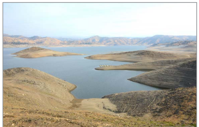
Millerton Lake is the reservoir on the San Joaquin River, and is drawn down in anticipation of the winter rains and spring snowmelt every year. In the fall of 2023, the reservoir was drawn lower than usual, so that the Friant-Kern Canal could be emptied and repaired, as the canal's capacity has been degraded due to land subsidence along its course because of groundwater pumping. CLUI photo
